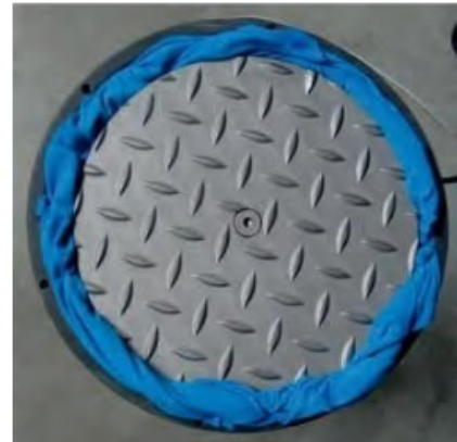
Figure 5.6 - Sealing the bollard
